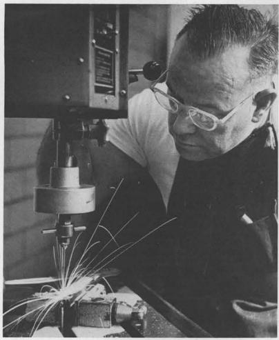
SPARKS FLY as John Moffet uses an electron drill to center drill a cylinder of alnico. The machine progresses at the rate of 1/2 inch every 11 minutes and is an extremely accurate machine tool.
